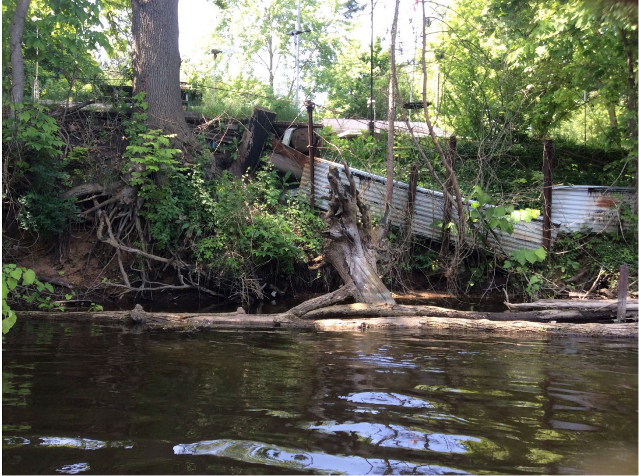
Figure 11. Site SJR09: Erosion along outside bend with roof of home in the background.
