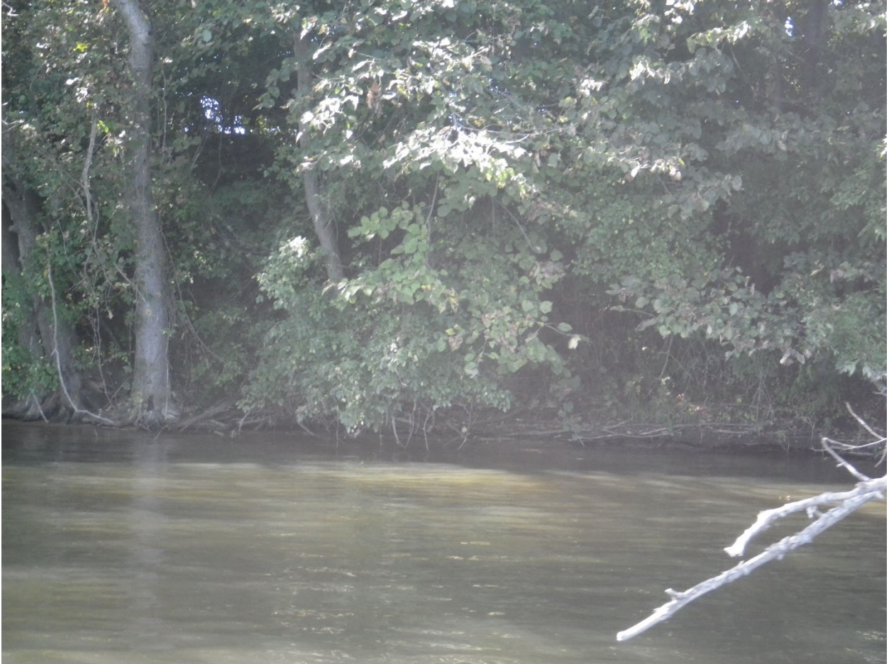
Figure 18. Site SJR16V2: Moderate erosion only due to the bank angle.
