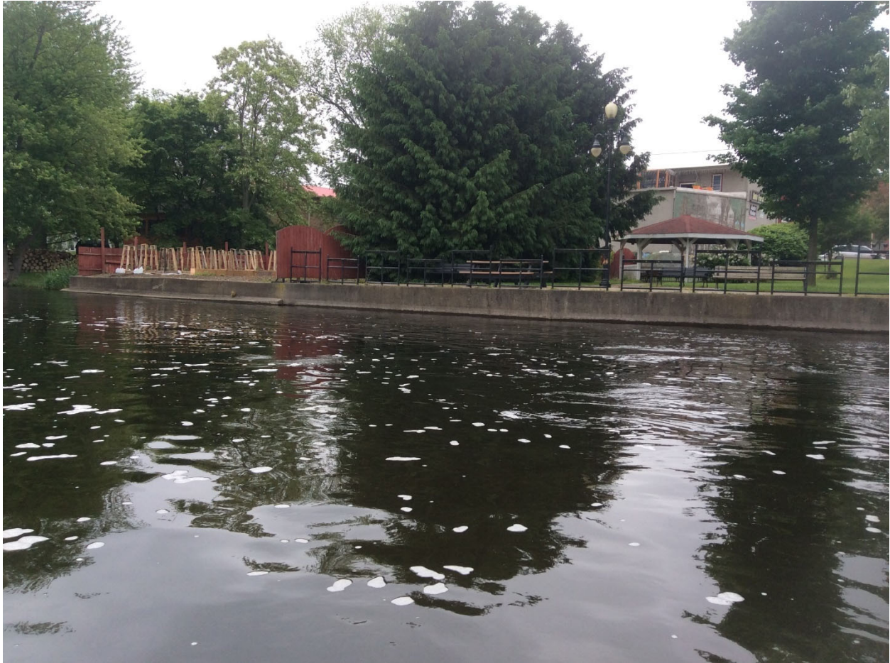
Figure 2. Site BA02: Example of shoreline armoring in the bypass reach area.
