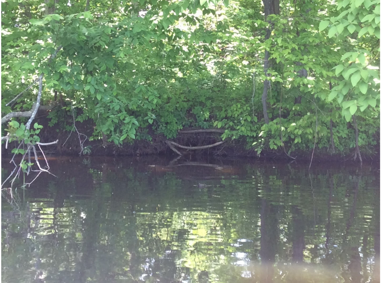
Figure 13. Site SJR15: Moderate erosion associated with an increase in bank angle.
