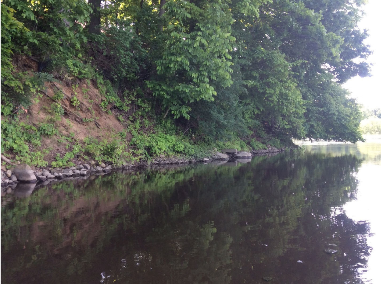
Figure 14. Site SJR18: Moderate erosion associated with an increase in bank angle and a decrease in root density.
