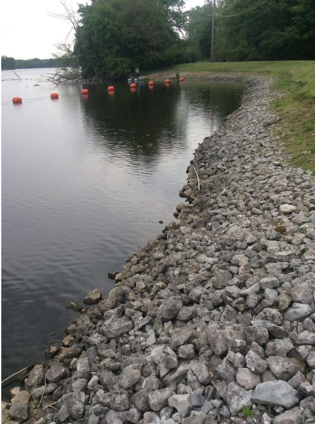
Figure 9. Site SJR45: Example of shoreline armoring.
