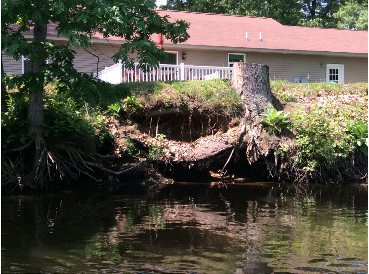
Figure 12. Site SJR10: Moderate erosion located along outside bend of river with home in background.
