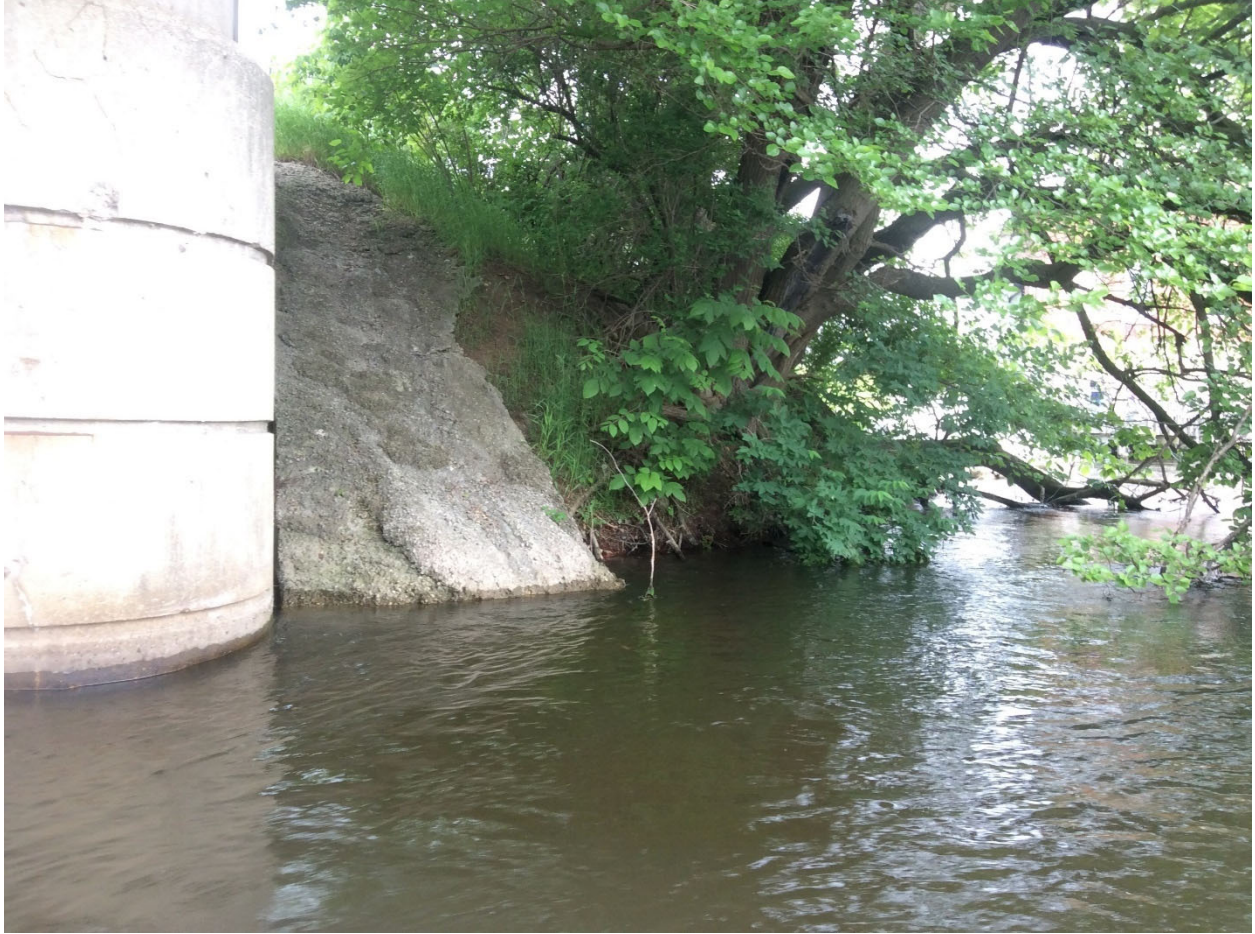
Figure 3. Site BA03: Area of Moderate erosion located at the Business Route US-131 Bridge.
