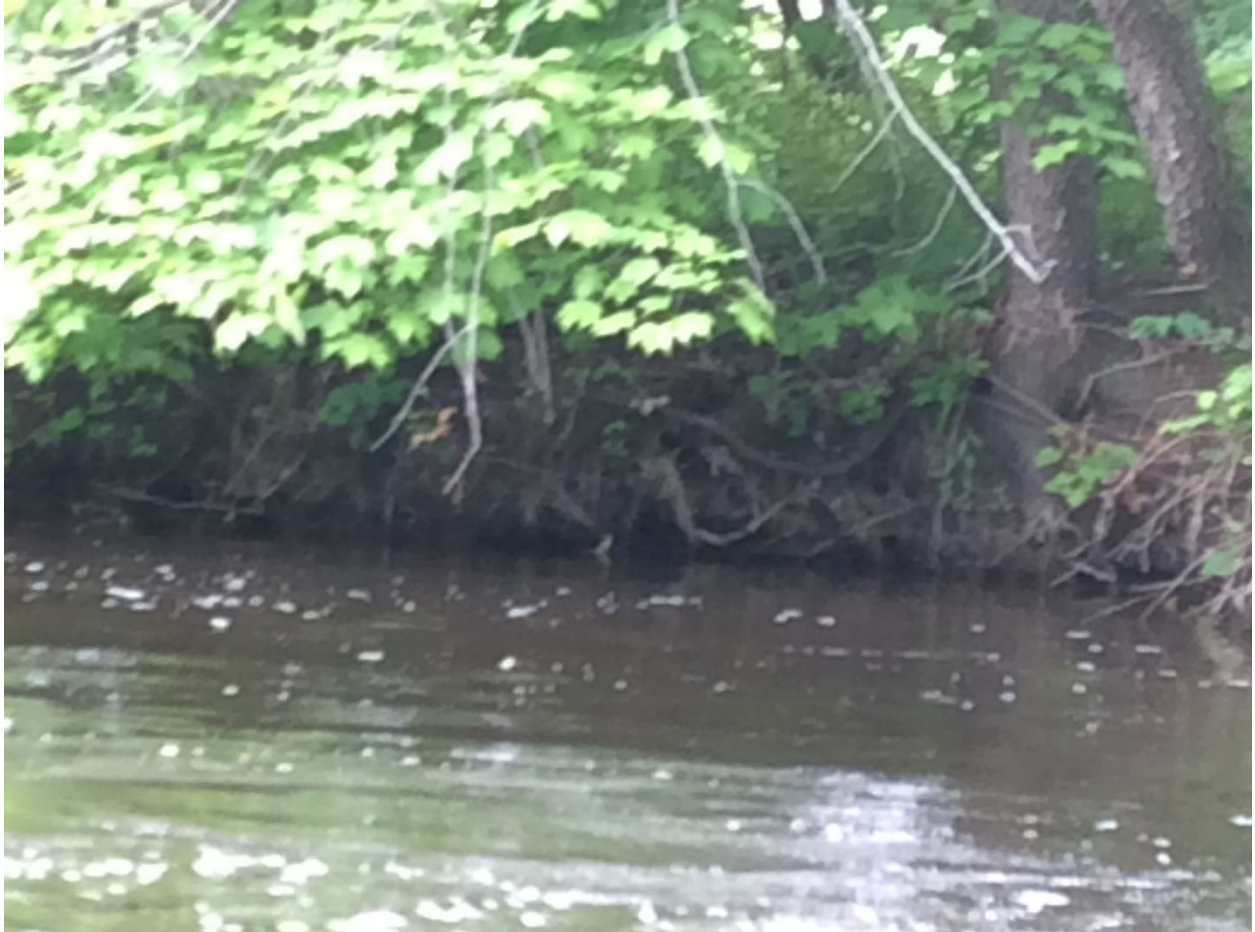
Figure 4. Site BA05: Moderate erosion near the water surface.
