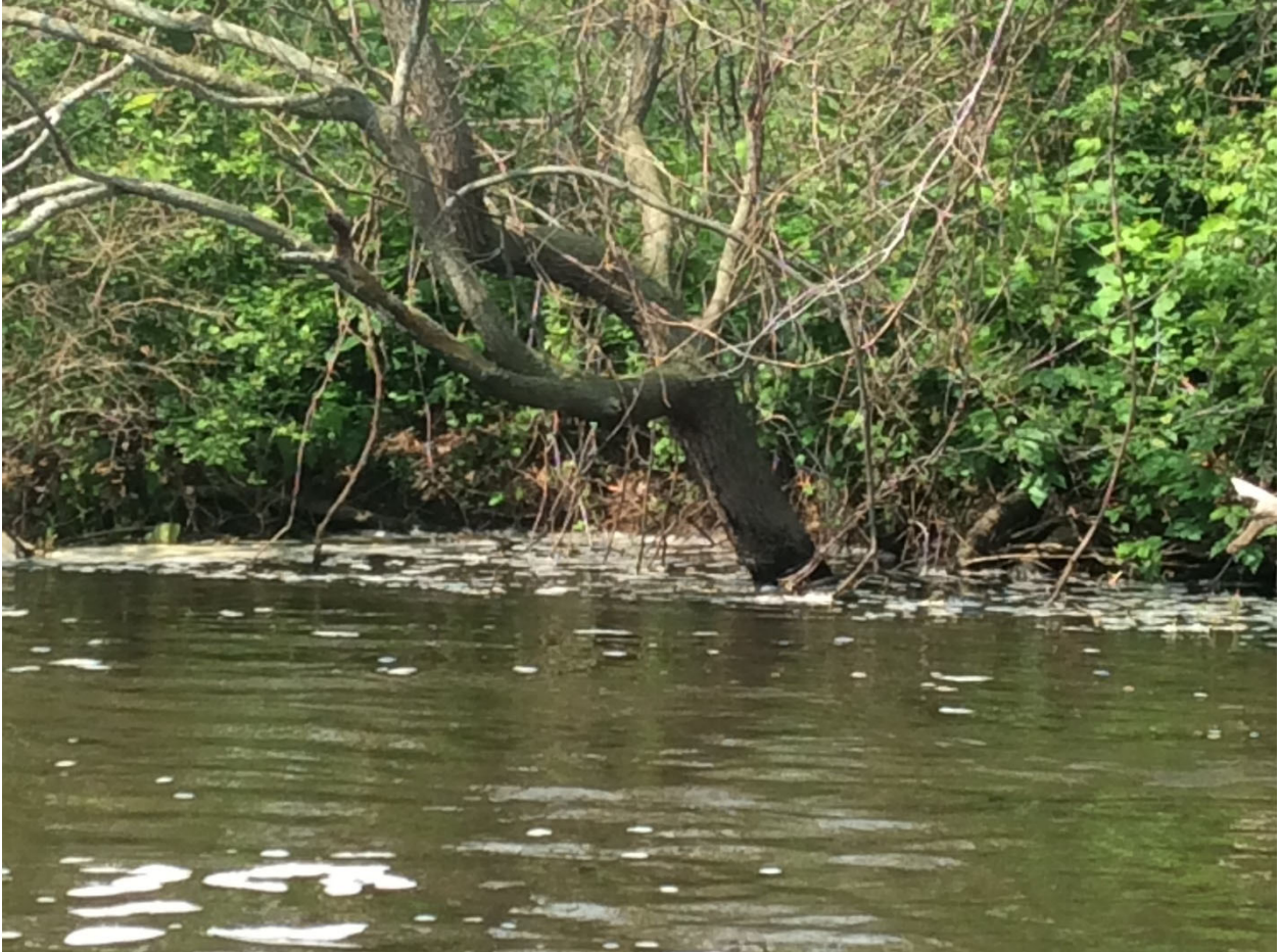
Figure 5. Site BA06: Moderate erosion near the water surface.
